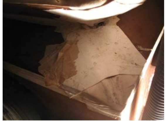
Figure 33: Unusual paper patch on a corner gusset.
