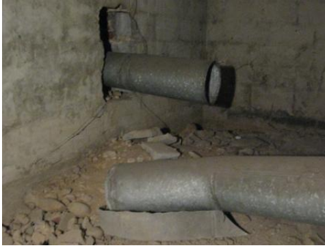
Figure 28: Former windlines under the chancel
