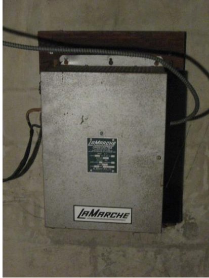
Figure 47: The rectifier under the choir.
