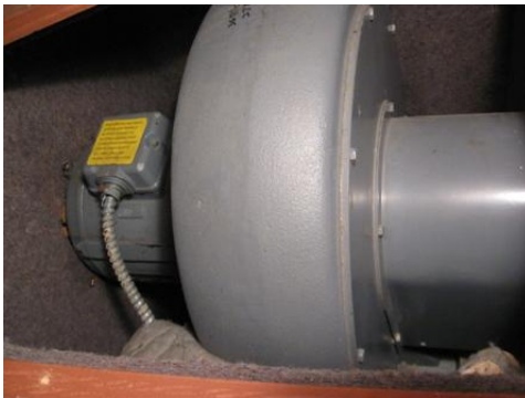
Figure 29: Meidinger blower in a muffler box lined with felt which is only partially effective in reducing wind noise.
