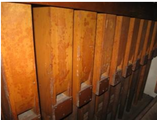
Figure 25: Bourdon 16 showing mold and mildew.
