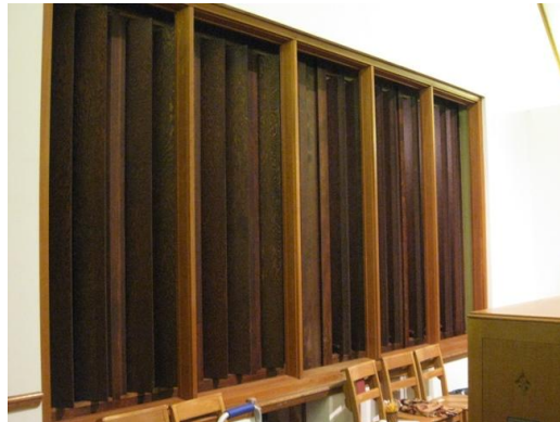
Figure 7: A view of the shades in their open position, allowing the full sound of the pipes to fill the church. By closing the shades, the organist can reduce the amount of sound that leaves the chambers.
